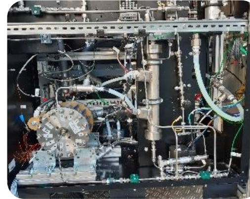
PEM Stack Test Bench
